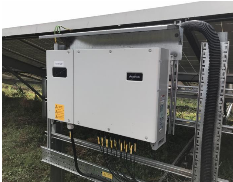
Photo 2-8: Typical string inverter (image reproduced courtesy of Huawei)
