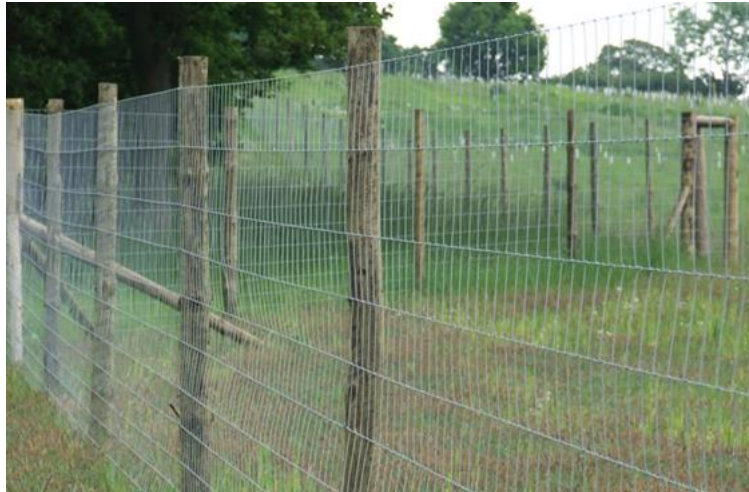
Photo 2-14: Typical deer security fence
